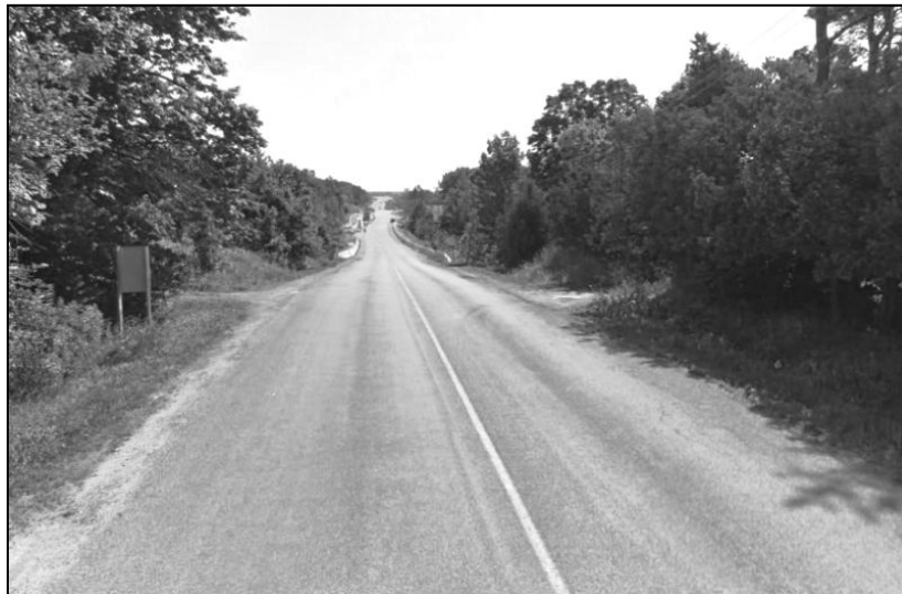
Figure 2. Teston Road Single Chip Seal as it Appears in 2011
