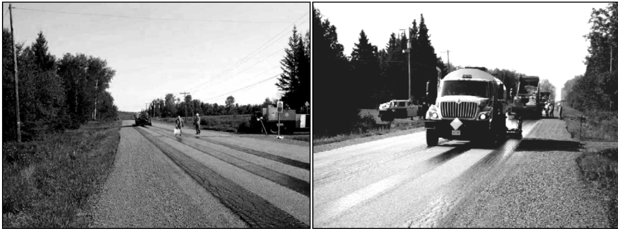
Figure 3. Construction of Highway 590 with the Use of Differential Spray Rate
