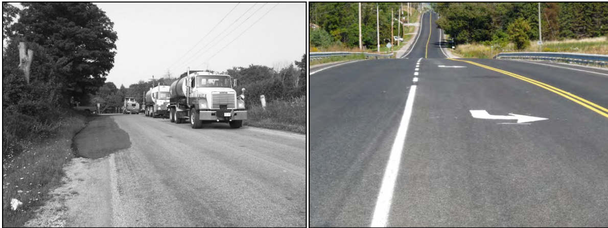
Figure 11. York Region Weston Road, Before and After Construction, 2009
