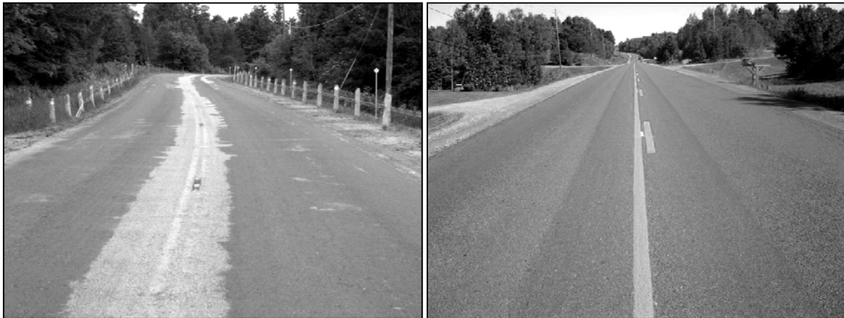
Figure 8. Illustration of Centreline Distress before and After Repair
