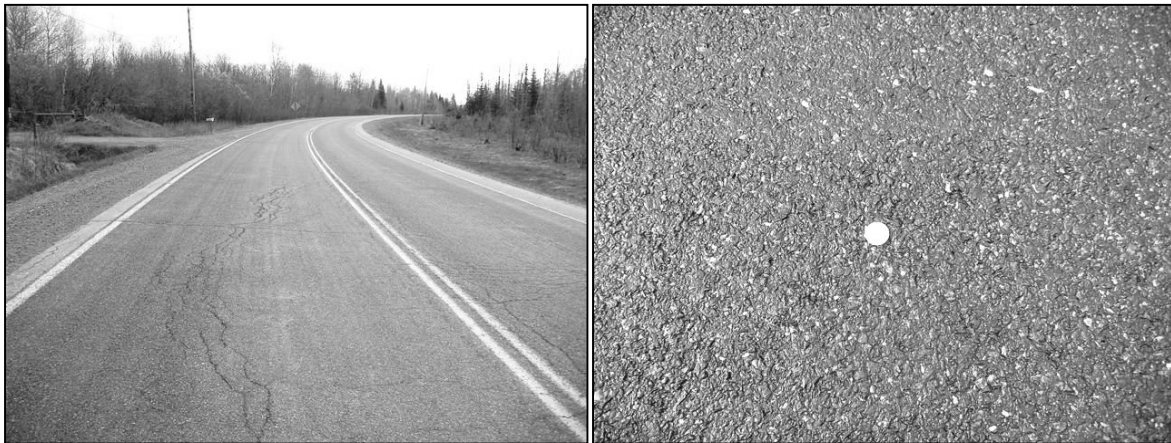
Figure 4. Typical Road Condition and Road Macrotexture for Highway 590 in 2011
