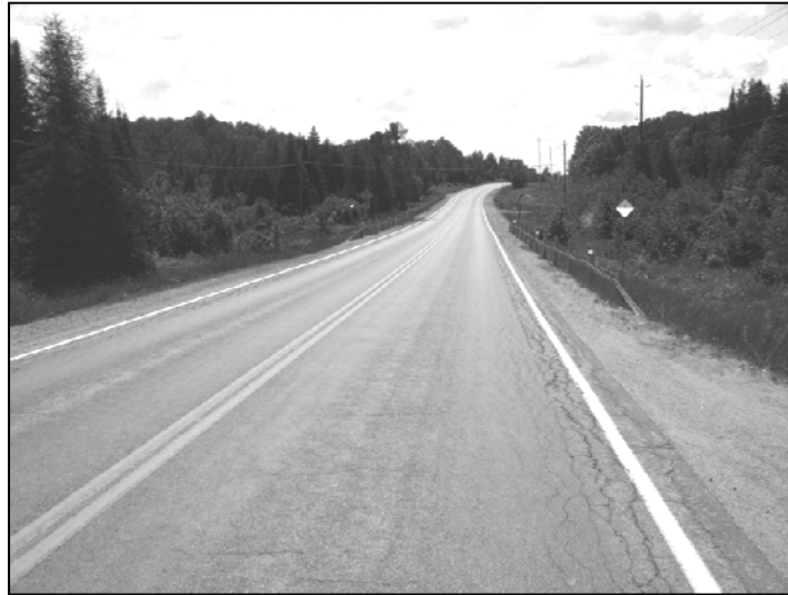
Figure 5. Illustration of Typical Pavement Condition in 2008 Prior to Construction
