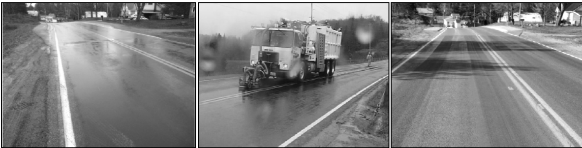
Figure 9. Illustration of Before, During, and After Water Blasting Treatment
