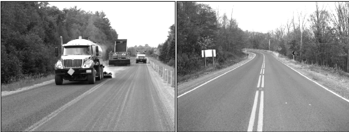
Figure 7. Illustration of Construction and Completed Double Seal Coat on Highway 28 in 2008
