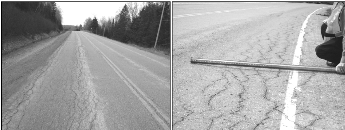
Figure 6. Illustration of Areas Requiring Hot Mix Asphalt Patching
