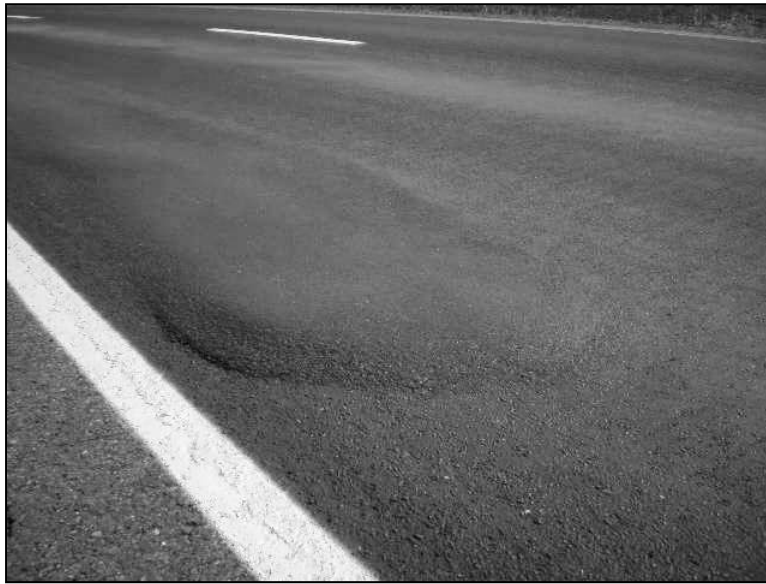
Figure 1. Illustration of Micro Surfacing Shoving
