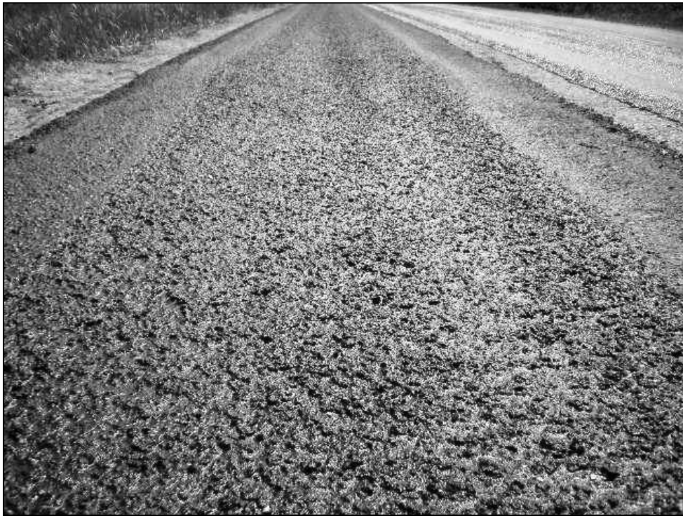
Figure 12. Texture of Micro Surfacing Rut Filling Before Top Coat
