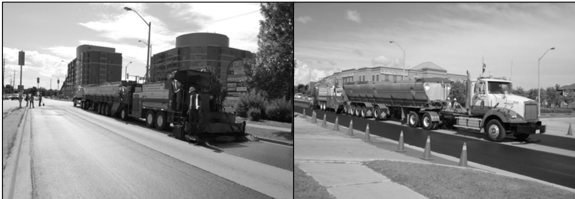
Figure 9. Continuous Mix Machine Working in the Town of Markham in 2008
