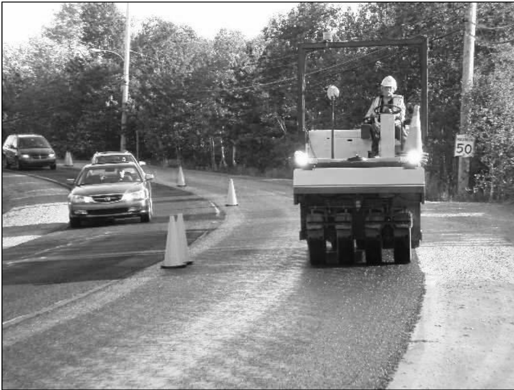
Figure 4. Rolling Micro Surfacing in Halifax for Smoother Finish
