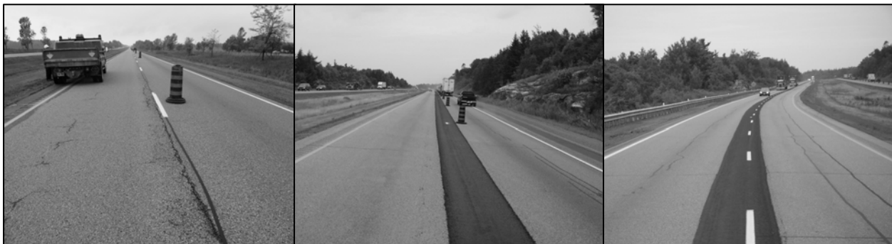
Figure 11. Highway 401 Centreline Micro Surfacing Application
