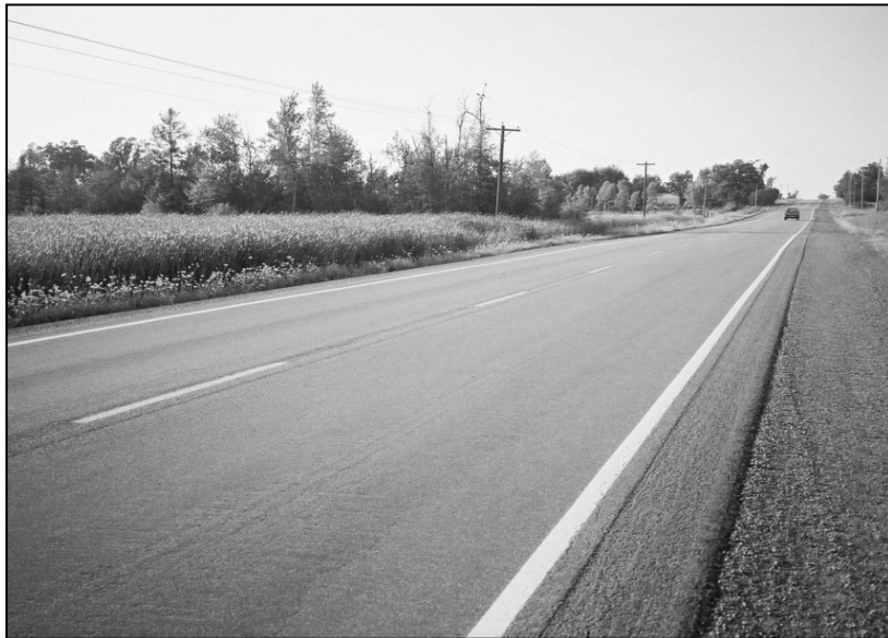
Figure 6. Completed Micro Surfacing on Highway 15
