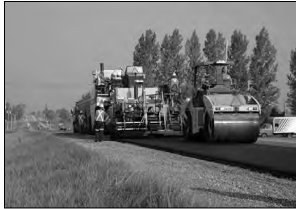
Figure 6b: Laydown of DAT
