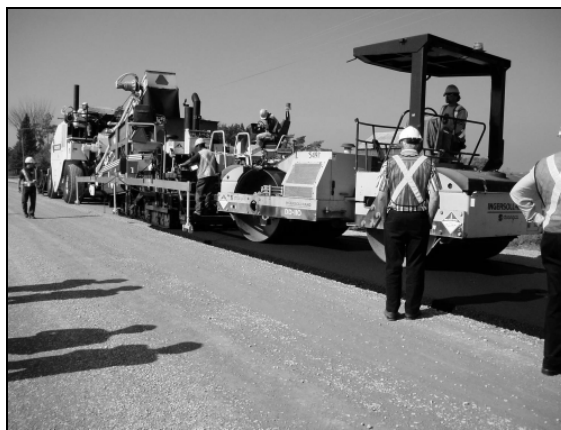
Figure 3b: Warm Mix Placement
