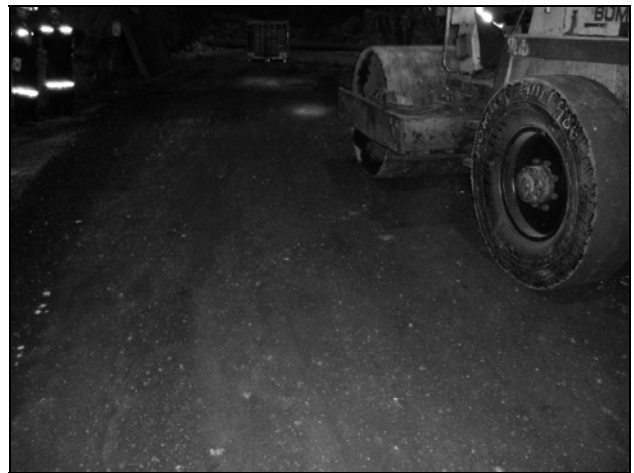
Figure 3b. Initial Compaction
