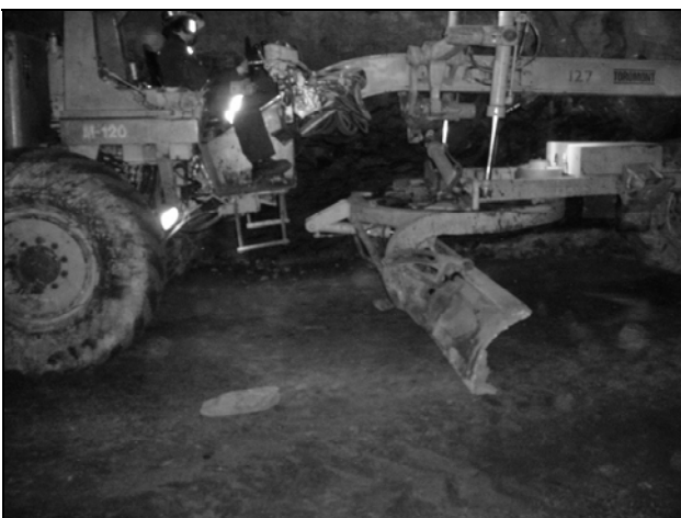
Figure 3c. Grading for Final Profile
