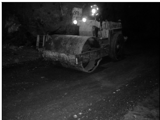
Figure 3d. Final Compaction of Surface
