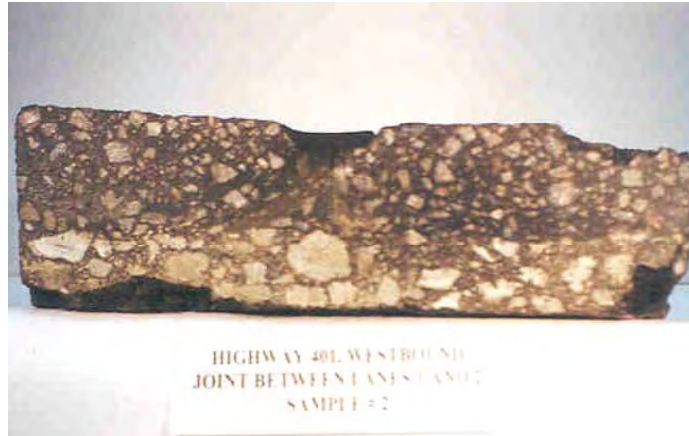
Figure 6. Cross Section of a Slab taken from Highway 401 Westbound in Mississauga
