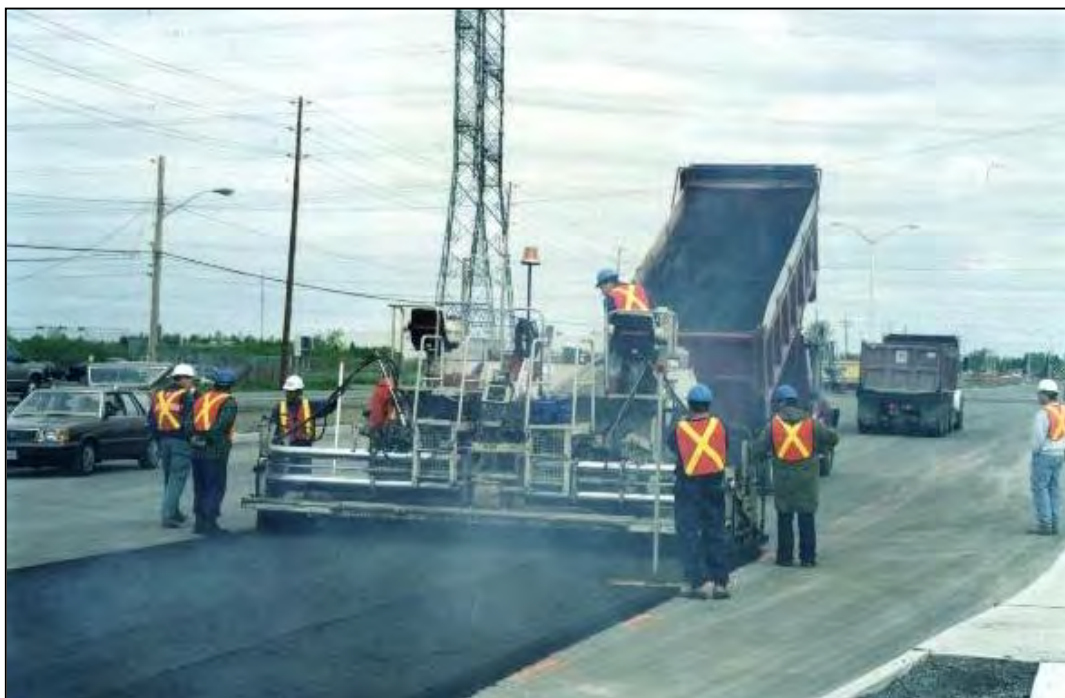
PHOTOGRAPH 3: Standard Asphalt Spreader Laying Performance-Graded Asphalt Cement Recycled Hot Mix
