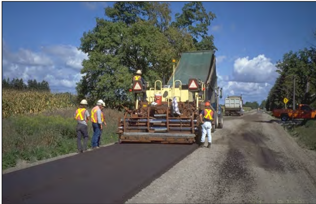
Figure 11 – Paving of Emulsion Stabilized Granular Material
