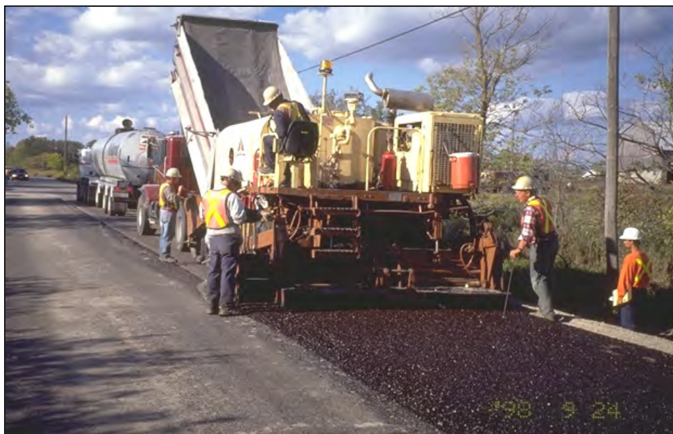
Figure 12 – Production and Placement of Open Graded Emulsion Mix using a Mix-paver
