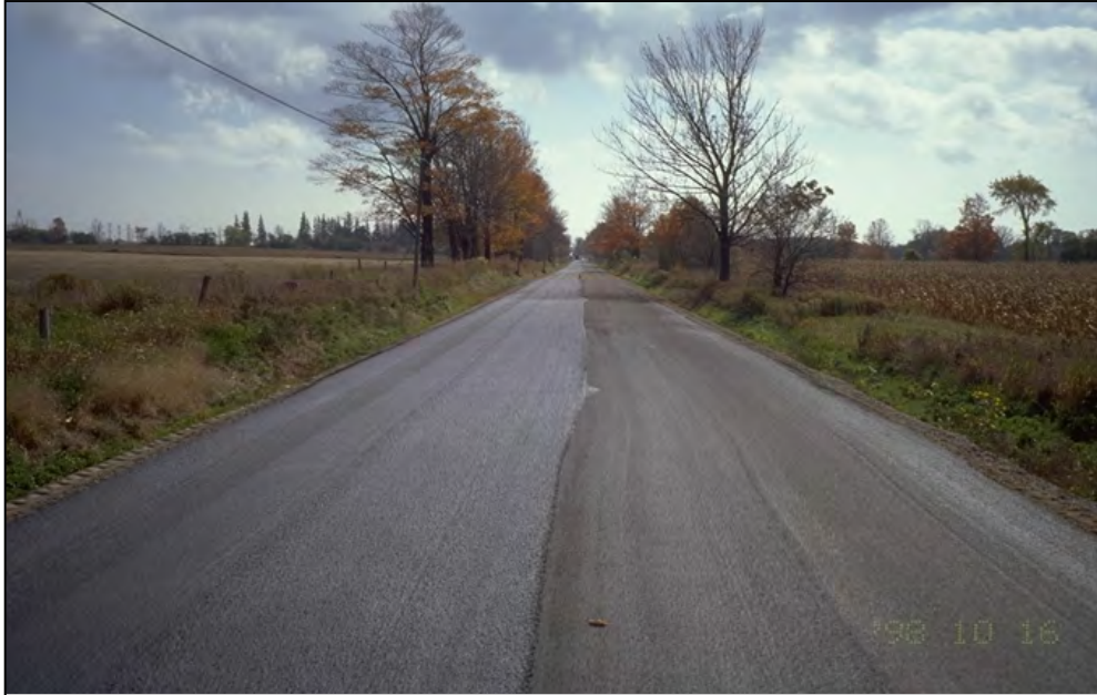
Figure 13 – Application of a Type II Slurry Seal Surfacing PERFORMANCE OF EMULSION MIXES
