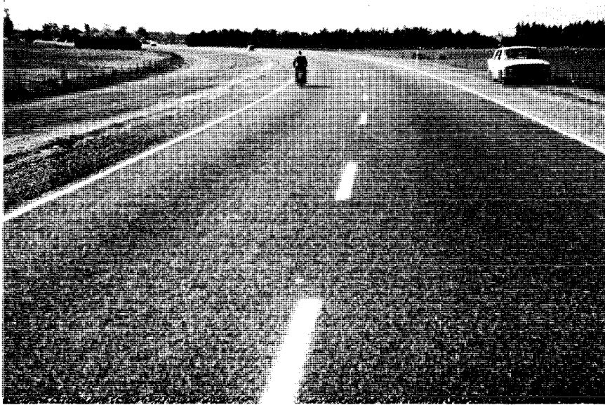
Fig. 4. New Zealand. Main Highway Taupo to Wellington. Double Surface Treatment on Consolidated Granular Base.
