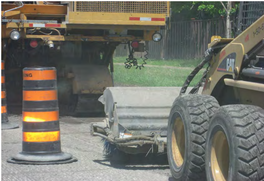
Figure 3. Sweeping the Milled Surface of Garth Street Prior to Warm Mix Asphalt Placement
