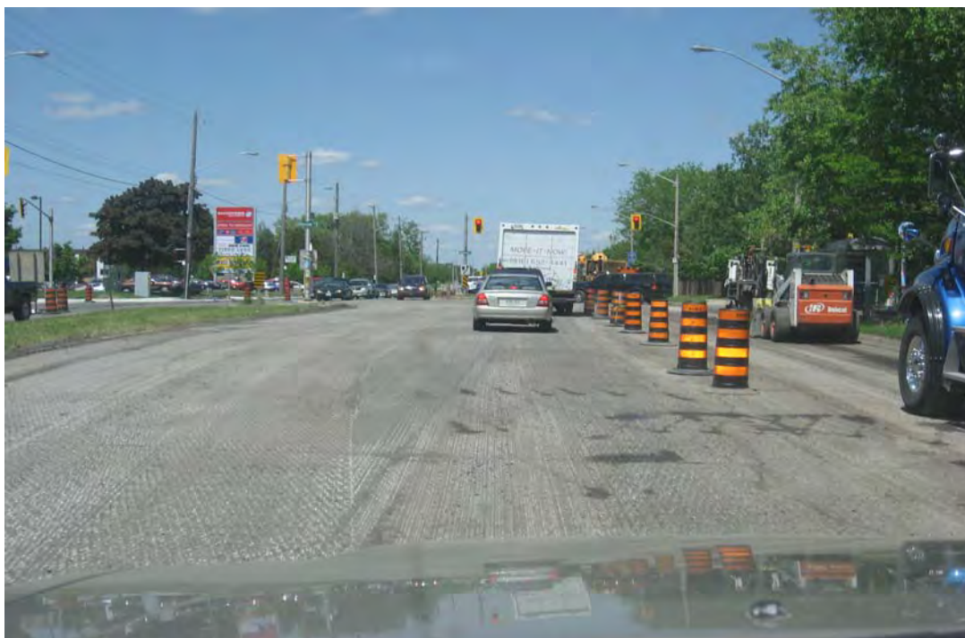
Figure 4. Garth Street – Prepared Milled Surface Prior to Warm Mix Asphalt Placement
