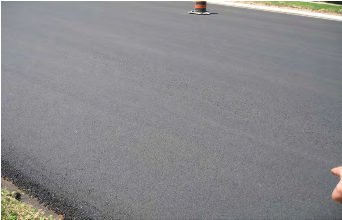
Figure 5. Warm Mix Asphalt (WMA) Mat on Garth Street, June 14, 2007
