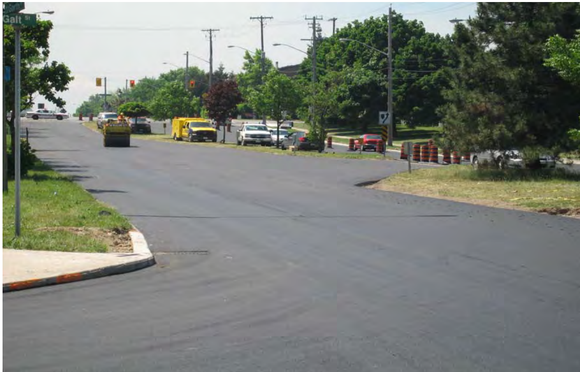
Figure 6. Warm Mix Asphalt (WMA) Mat on Garth Street, June 14, 2007
