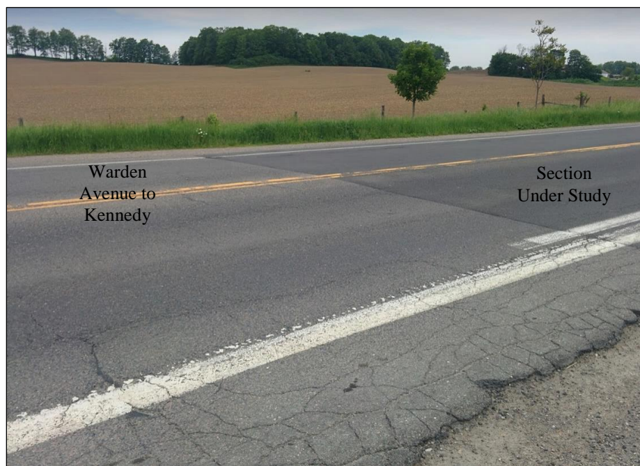
Figure 14. Comparison of the study section to an adjacent section that exhibited more distresses for nearly the same service life.
