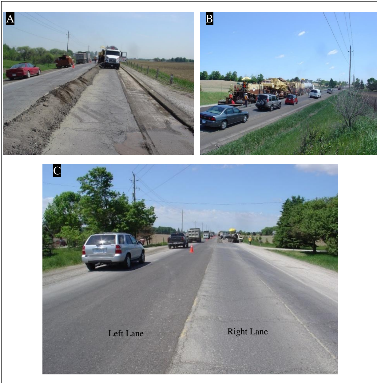
Figure 4. (A) A Section Milled by Small Milling Machine and Resultant Windrow, (B) Illustration of Cold-In Place Recycling Train, and (C) Completed CIR mat prior to Hot Mix Asphalt Paving
