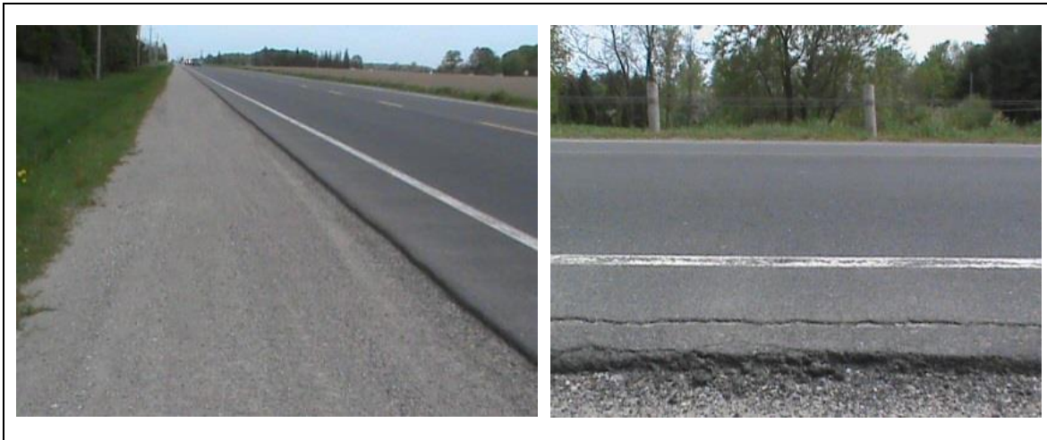
Figure 13. Typical Shoulder Condition of Bloomington Road
