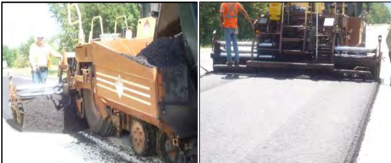
Figure 8. Placing Rubber Asphalt Warm Mix
