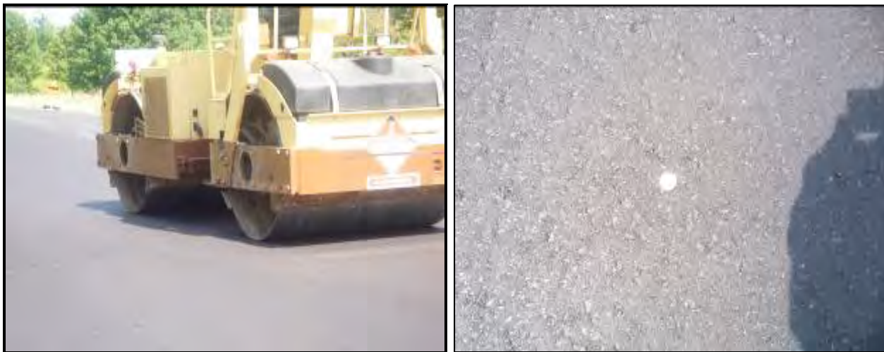
Figure 10. Rubber Asphalt Warm Mix Finished Mat
