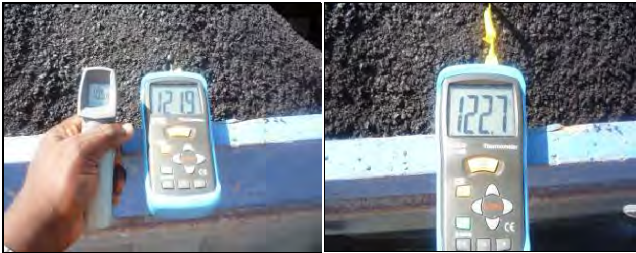
Figure 5. Rubber Asphalt Warm Mix Temperature during Hauling
