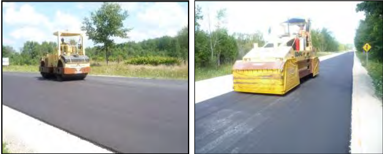
Figure 9. Rubber Asphalt Warm Mix Breakdown and Intermediate Rolling
