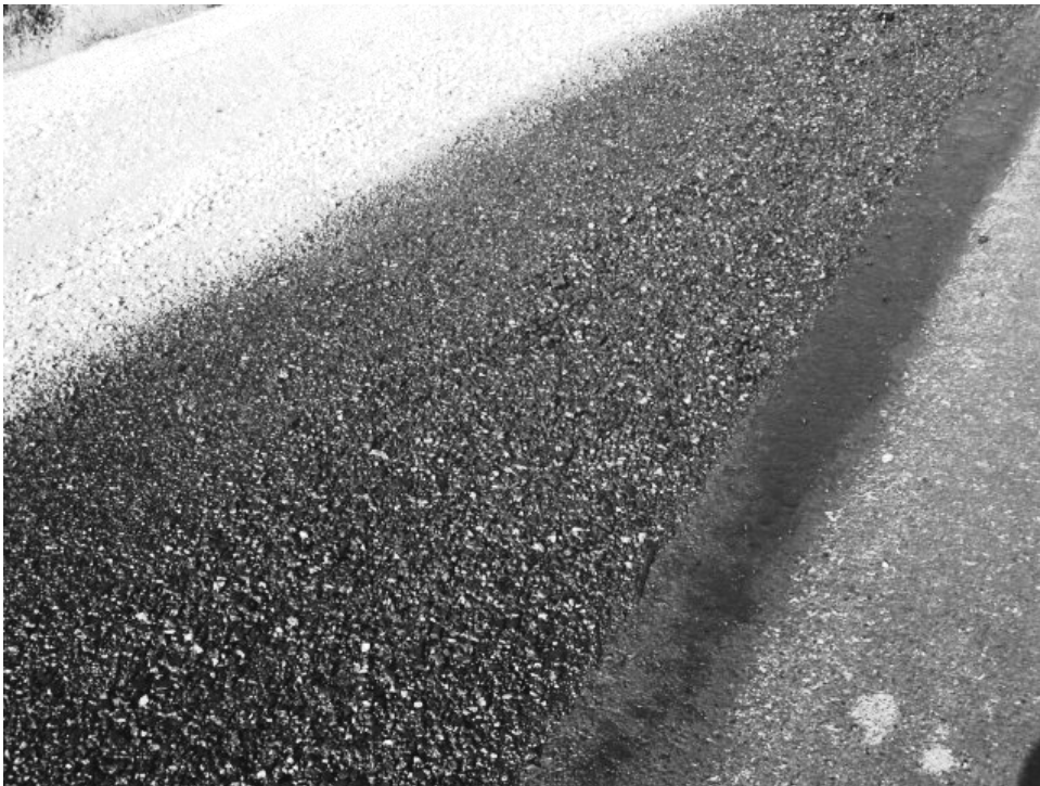
Figure 14. Granular Shoulder Sprayed with Solvent-Free Emulsion Prime
