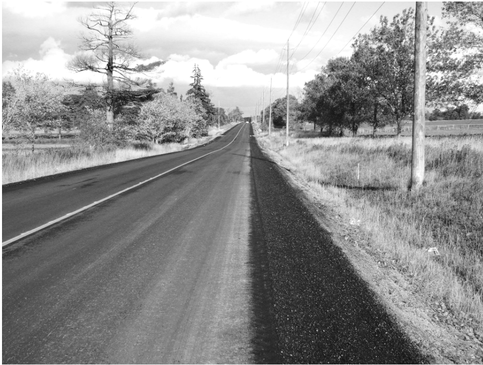
Figure 13. King-Vaughan Line after Shoulder Priming with Enviroprem Emulsion
