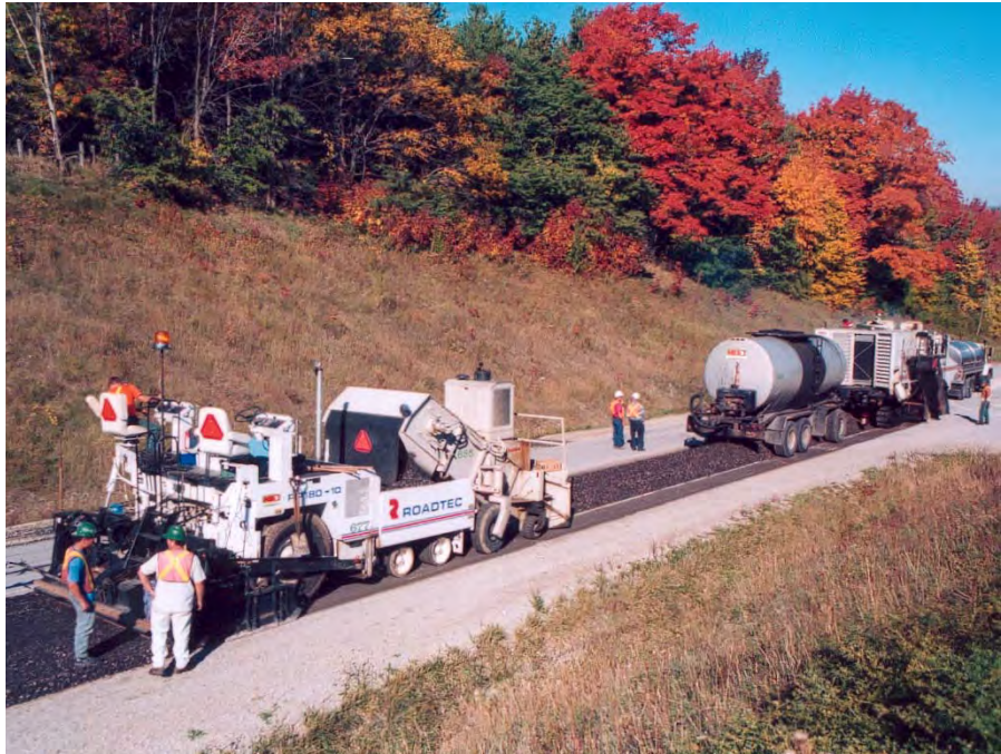
Photograph 2: Single-unit recycling train with placement using a standard paver
