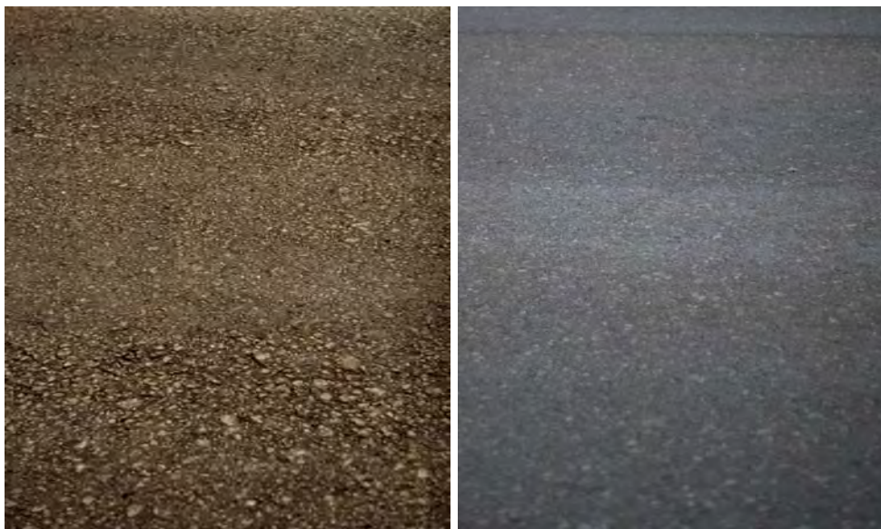
Photograph 6: Segregated mat vs segregation free mat
