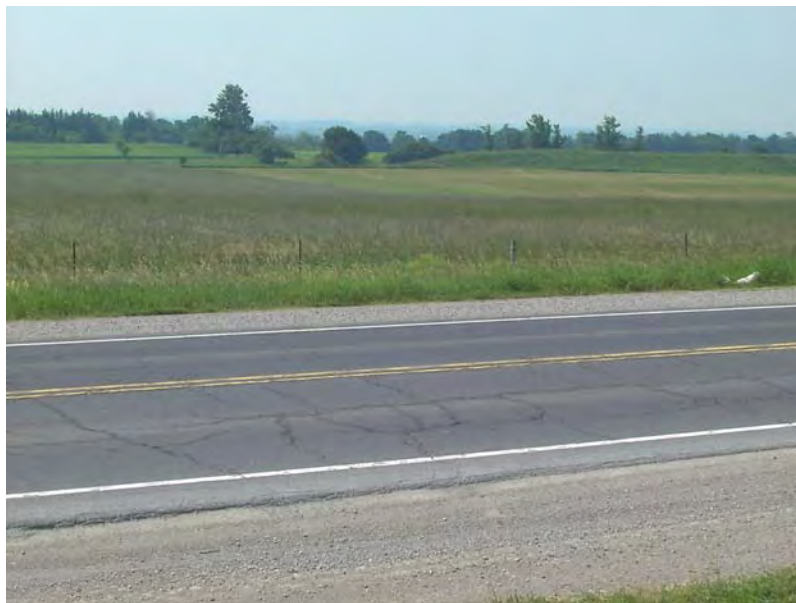
Photograph 1: Well drained structurally sound candidate for Cold In-place Recycling
