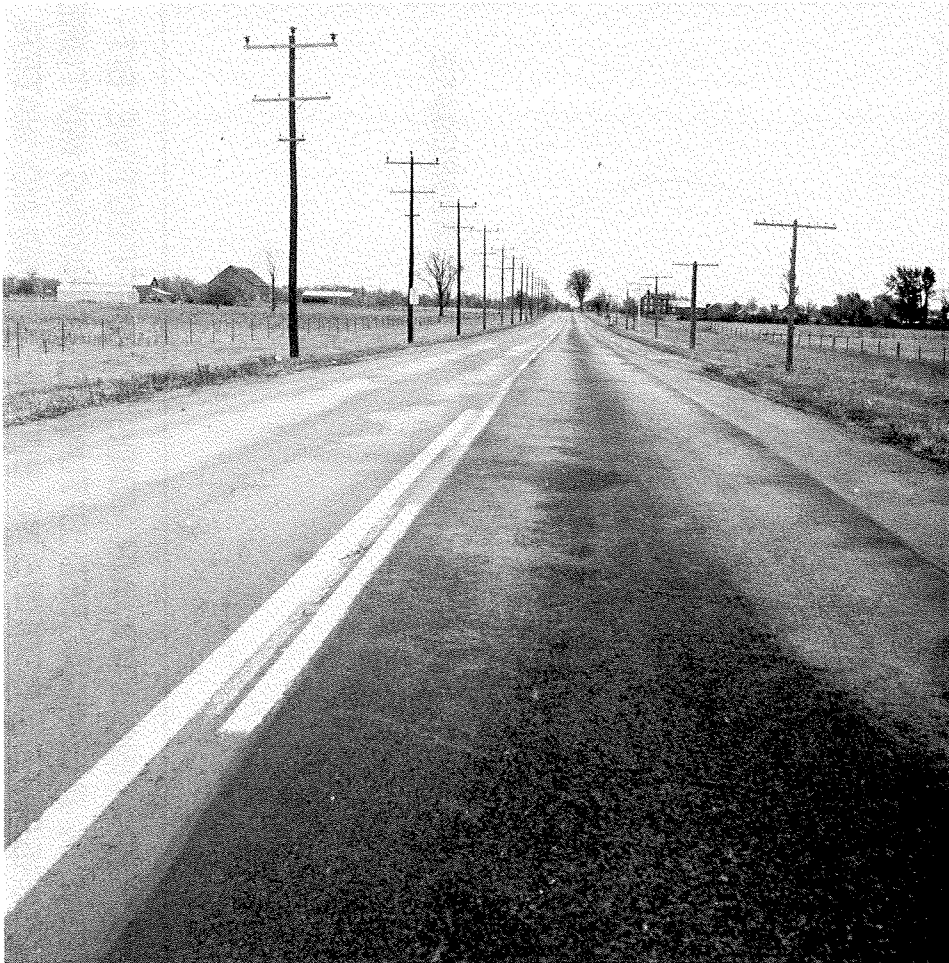
Fig. 9 Illustrating The Futility Of Trying To Cure A Flushed Or Bleeding Asphalt Pavement Condition By Burning Off The Asphalt That Has Oozed Out Onto The Pavement Surface.
