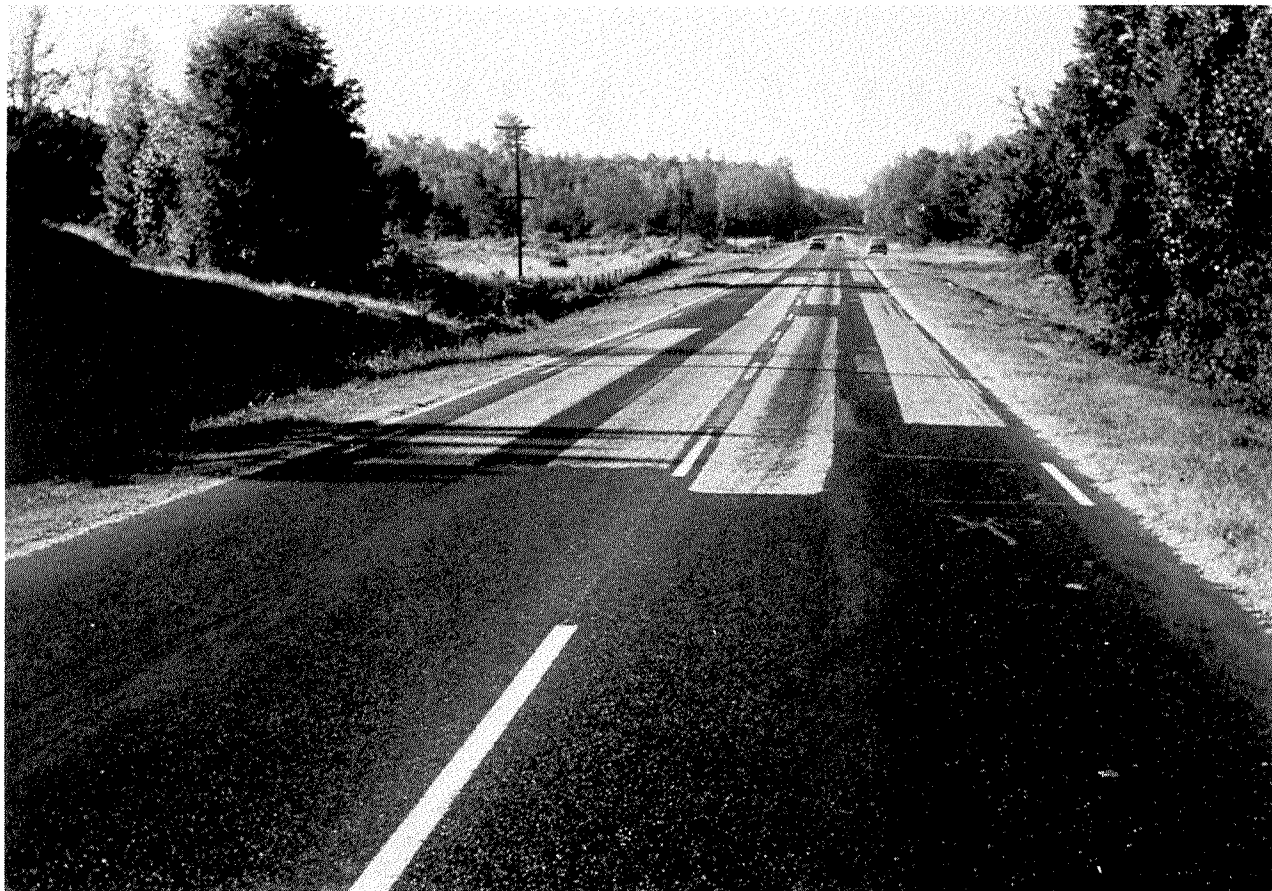
Fig. 1 Badly Ravelled Pavement Due To Serious Underasphalting
