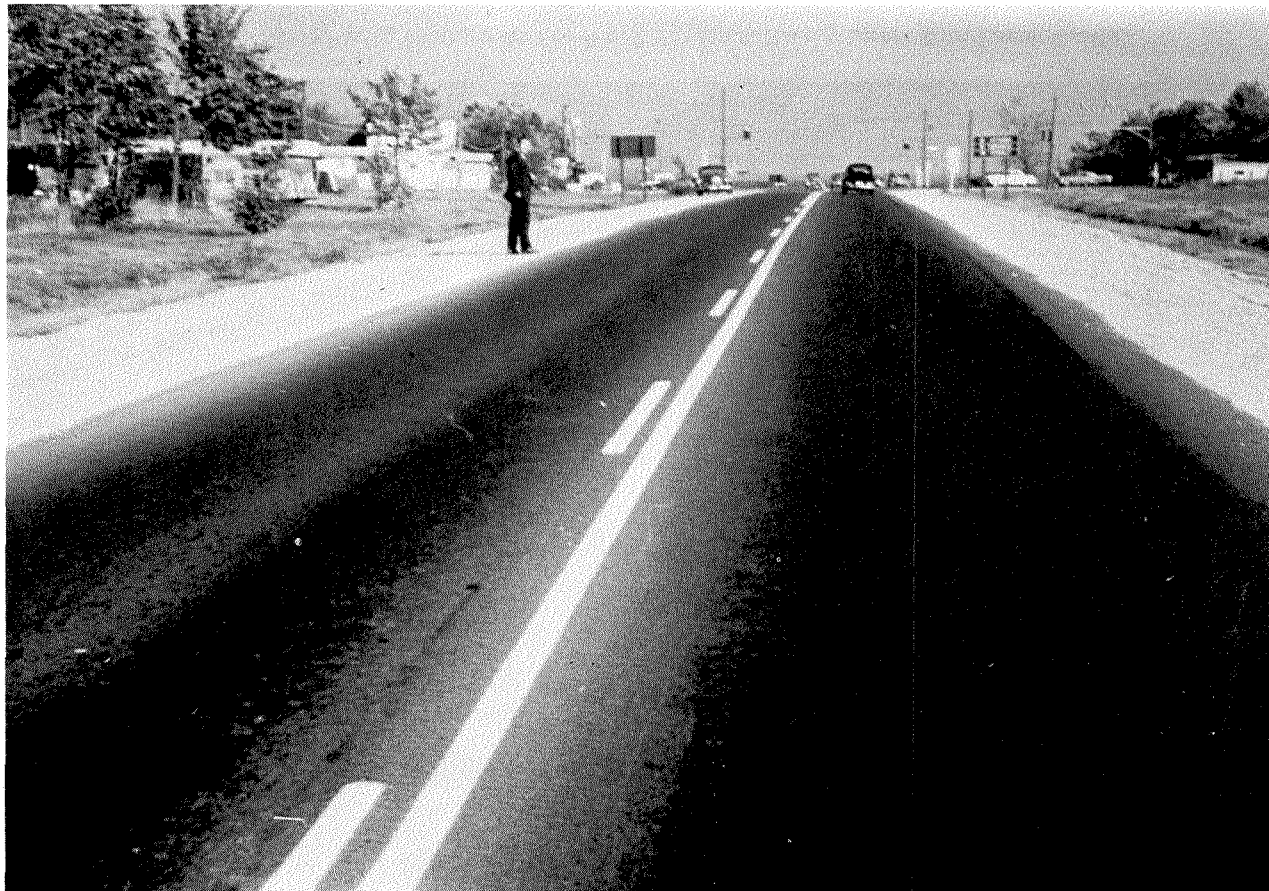
Fig. 2 Serious Flushing Or Bleeding Due To Excessive Asphalt
