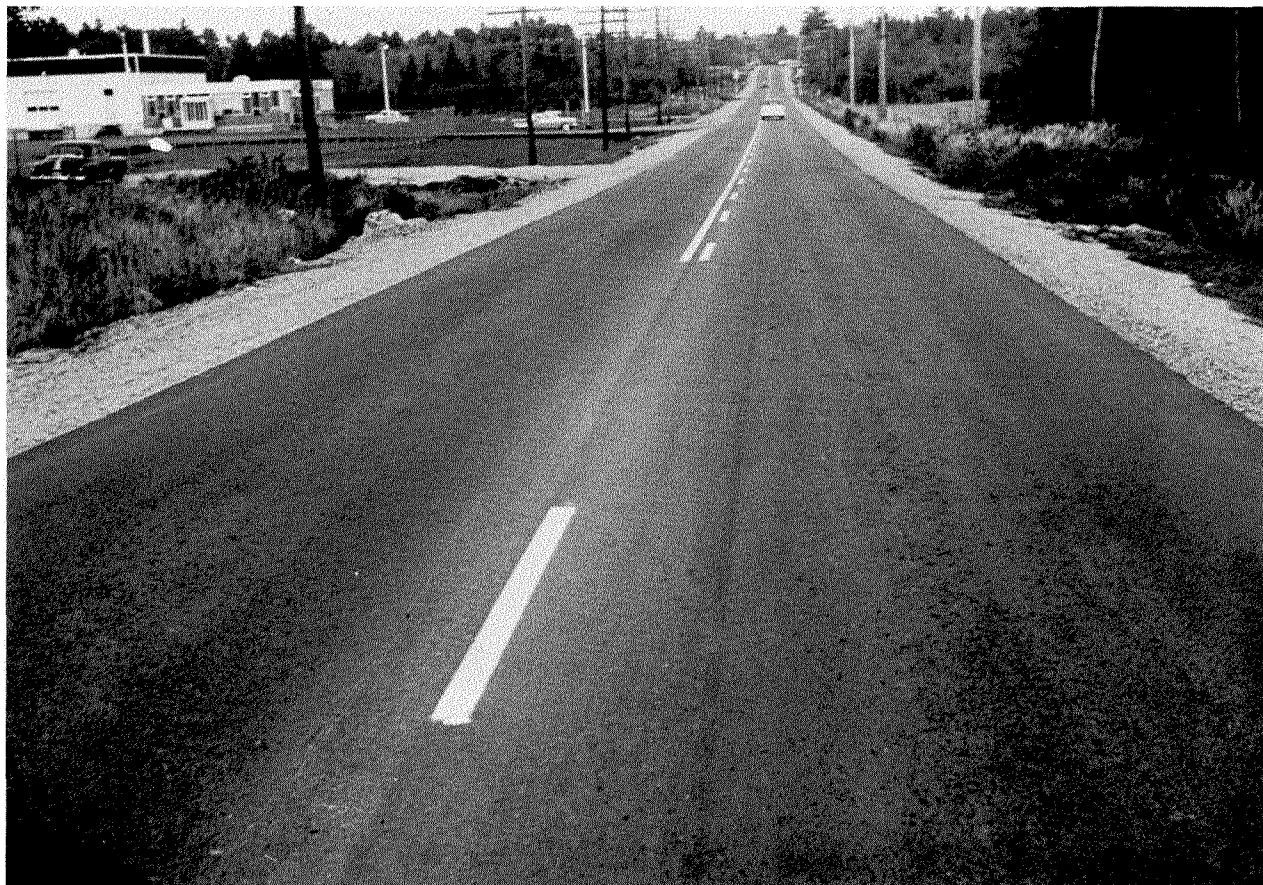
Fig. 3 Same Paving Mixture As For Fig. 2 But On A Nearby Street With Lower Traffic Volume
